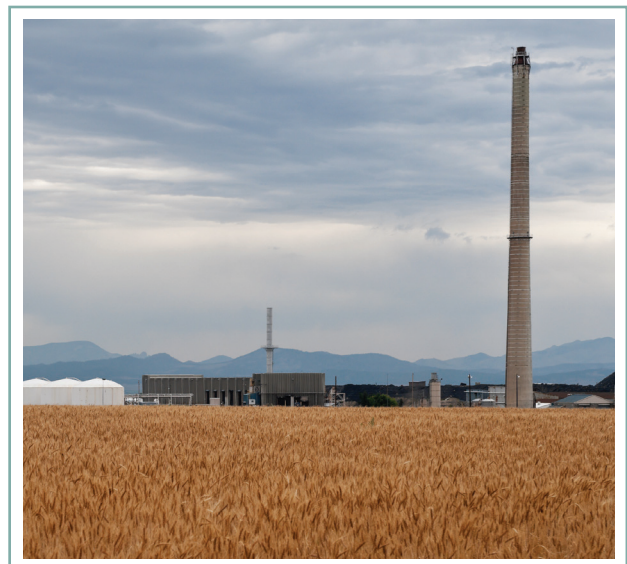
The East Helena smelter, a Superfund site, in Montana before scheduled demolition. Photo: Ron Armstrong/Getty Images
