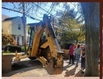
Municipal contractors actively replacing clay pipes with newer, sturdier PVC pipes.
